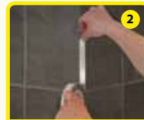
2 Apply revealed tape to wall
